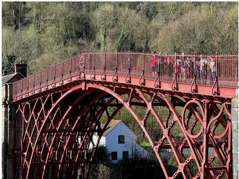
The fans at Bridgecon
