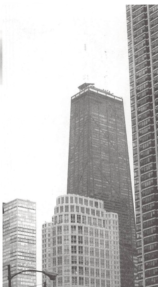
John Hancock Building
