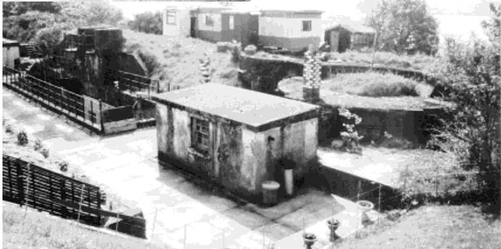
Portkil 6-inch Battery (Ian Stevenson)
