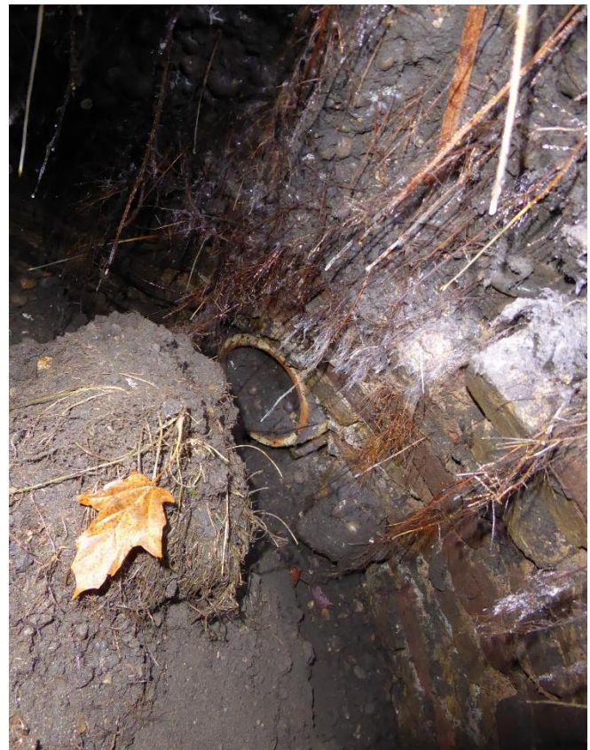
Inside of brick structure looking downwards; view of curved brick walls and the ceramic pipe
