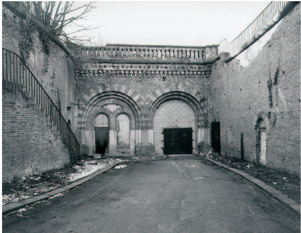
Figure 27 The Inner Entrance, showing the road tunnel and the guard room; the blocked doorways on the right flank wall lead to the water tanks (NMR: AA00/9818)
