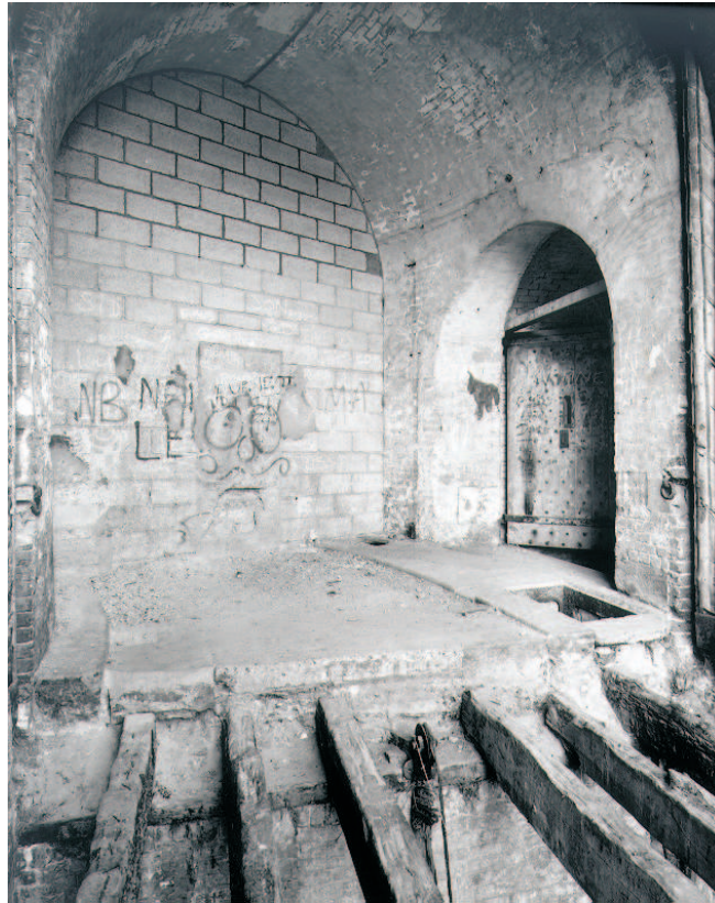
Figure 21 The blocked road tunnel and doorway to the postern gate, with the remains of the bridge in the foreground (NMR: AA00/9840)
