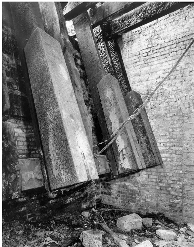
Figure 17 The counterweight recess with the bridge counterpoise weights in position (NMR: AA00/9846)
