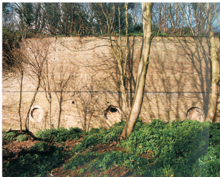
Figure 33 The scarp revetment of South Entrance Ditch in 1999, showing how the infilling of South Entrance Ditch has sealed the embrasures and loopholes. The smoke vents remain visible but blocked (NMR: AA00/8595)
