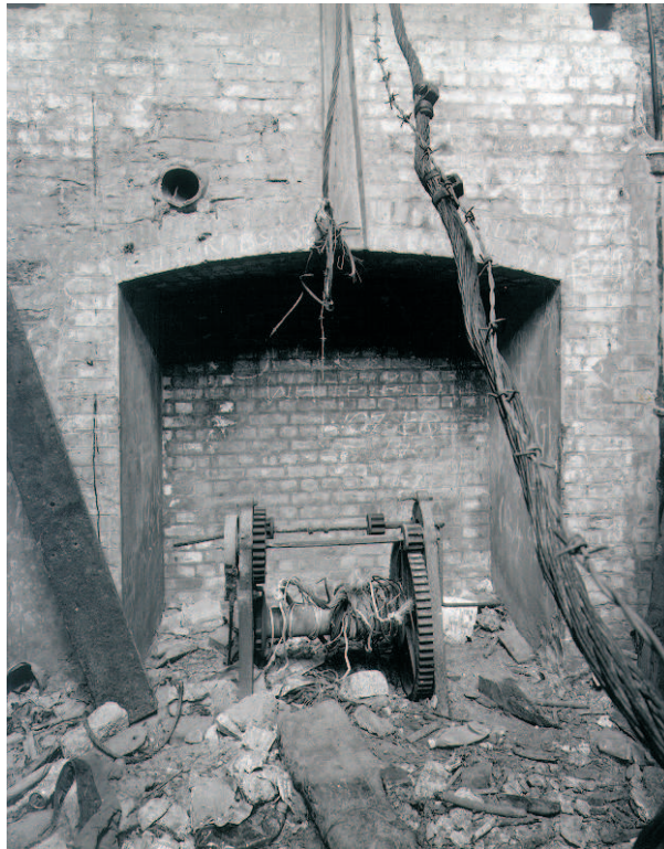
Figure 18 The winch in the counterweight recess (NMR: AA00/9847)
