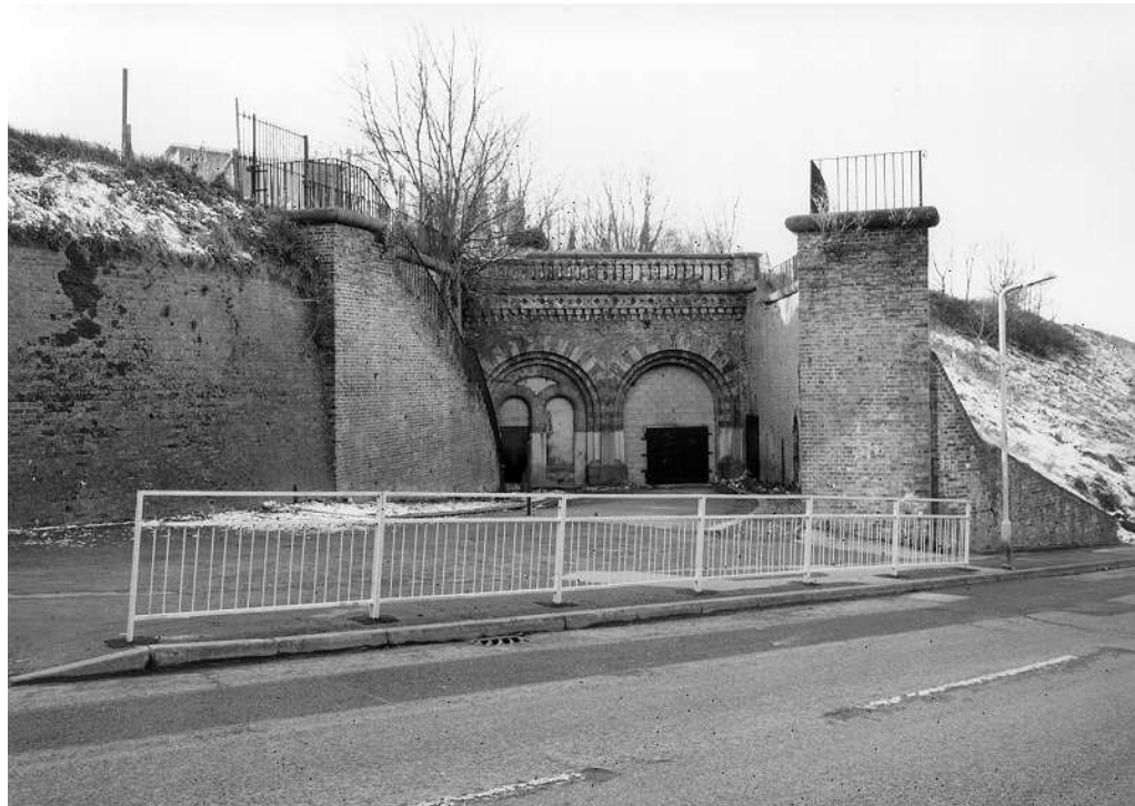
Figure 30 The Inner Entrance, showing the new route of the Centre Road which by-passes it (NMR: AA00/9815)
