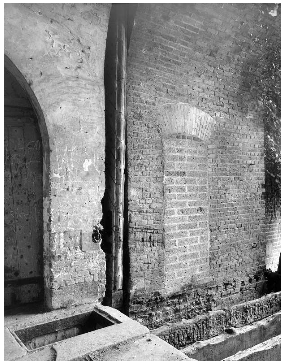
Figure 20 The blocked doorway to the winch room, with the remains of the bridge in the foreground (NMR: AA00/9842)
