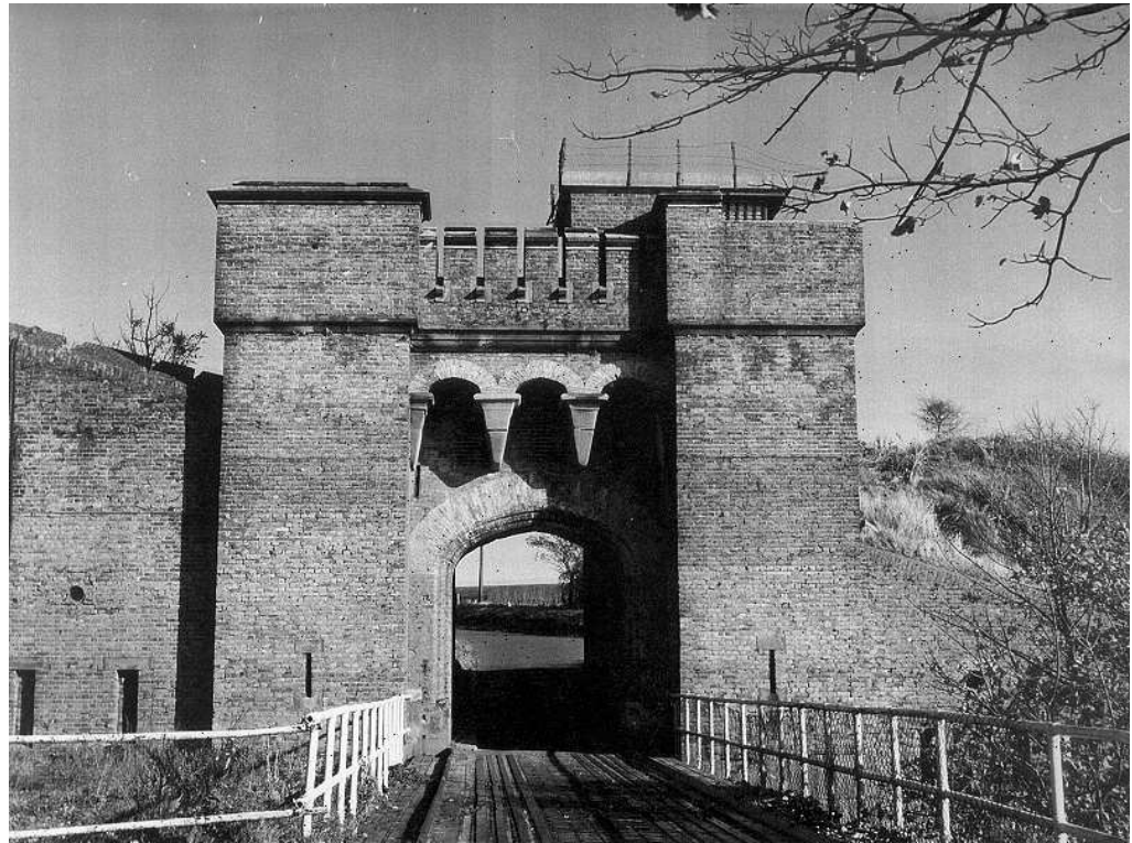
Figure 35 Archcliffe Gate in 1959, showing the Second World War observaton post on top (NMR: A.5513/5)
