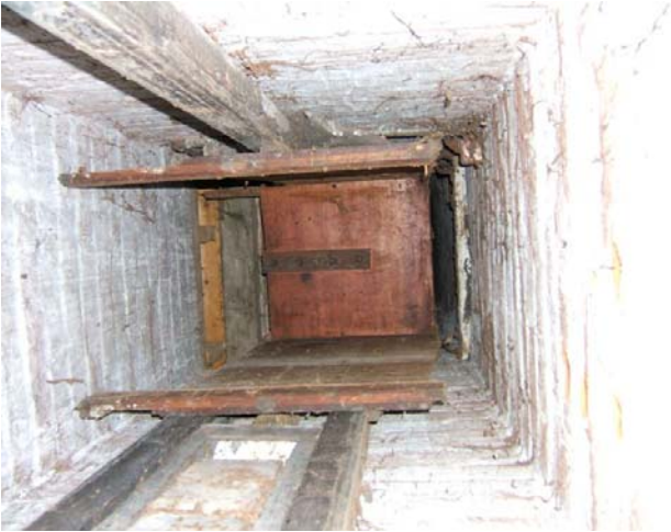
Image 81: Interior of dumb waiter looking upwards.
