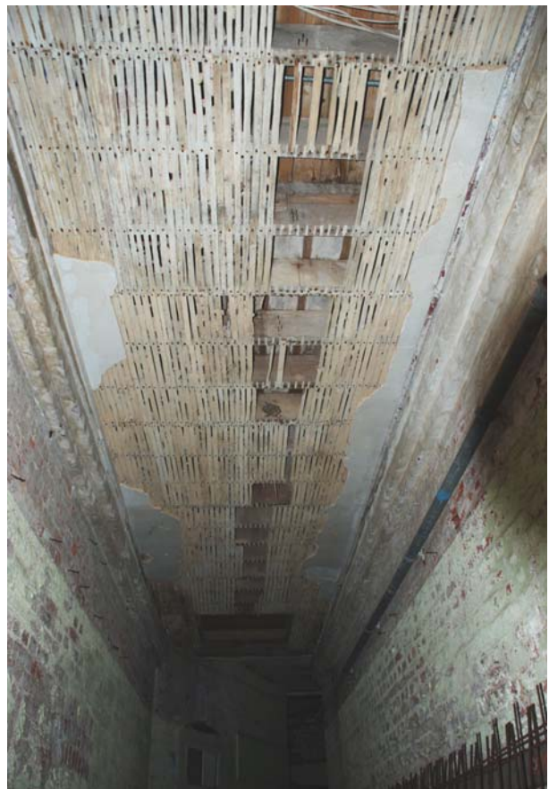
Image 08: Original ceiling: lathe and plaster.
