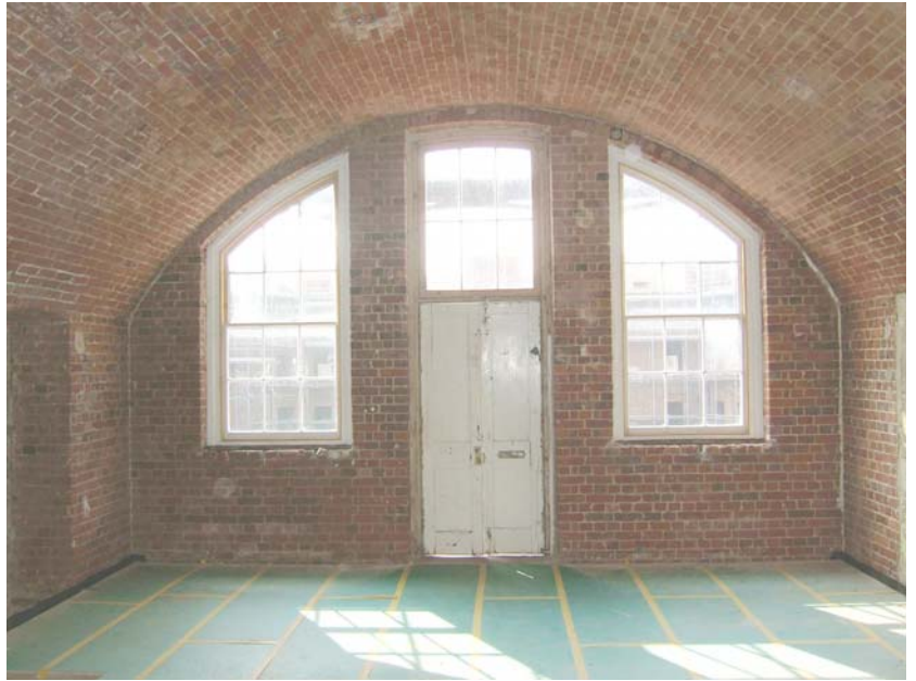
Image 16: Interior of barrack room looking towards interior of the fort. Sash windows and double door. Vaulted brick ceiling.
