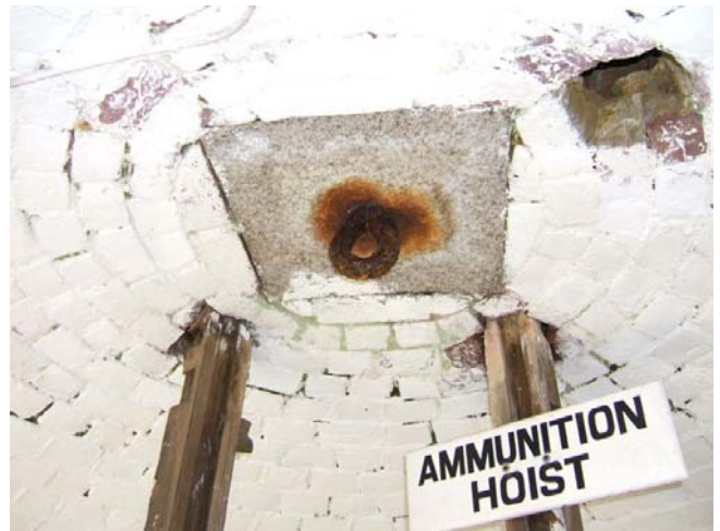
Image 78: View of the top of ammunition hoist showing iron ring for hoist tackle.
