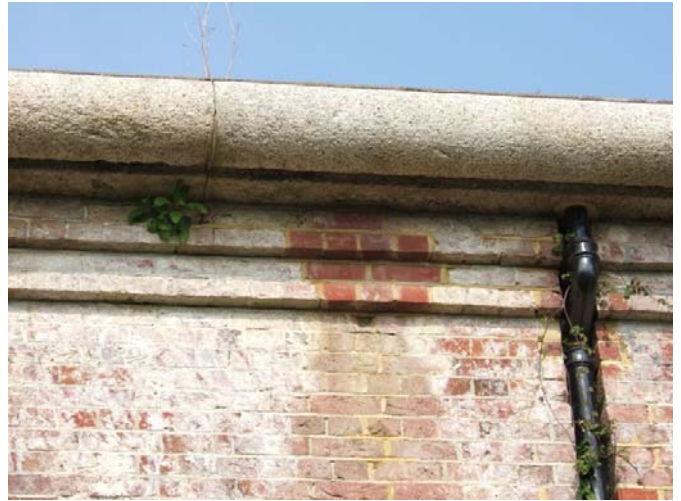
Image 82: Outside cornice showing granite coping stone with downpipe.
