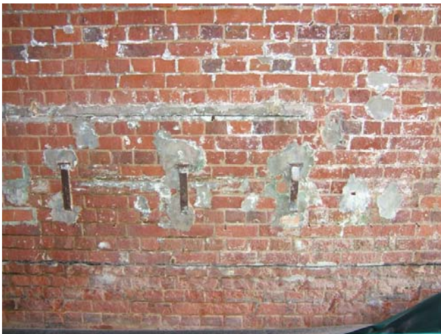
Image 49: Fittings for wash sinks and bitumen sealing lines.
