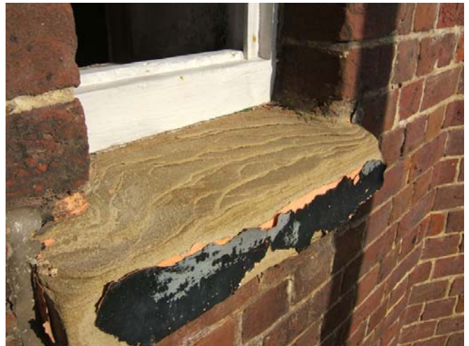
Image 56: Weathered window sill on first floor.
