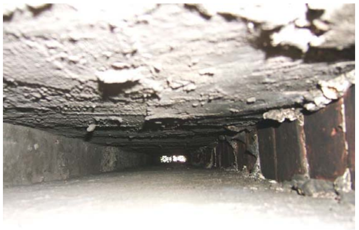
Image 18: View along air vent from interior of building to the exterior metal covering, as seen in image 20, to the right of the gauged brickwork of window flat arch. This vent originates in base of fireplace as in image 22.
