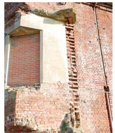
Image 36: Detail of upper storey: brick scars and concrete roof remnants.
