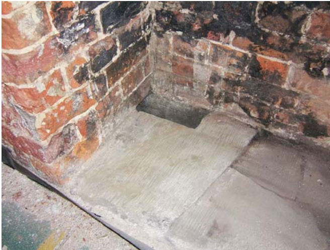
Image 19: Opening of air vent in base of fireplace.
