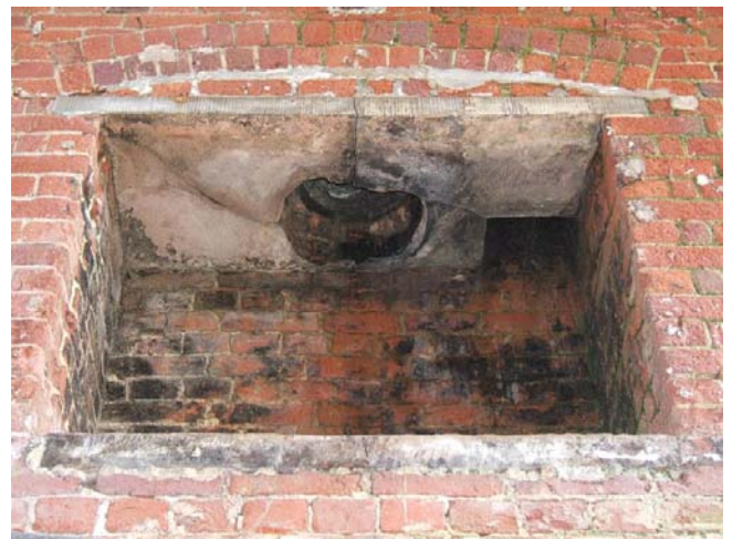
Image 22: View upwards into another altered fireplace showing the two shaped sandstone lintel pieces, formed to accommodate the flue of a stove. To the right can be seen the upper vent of ventilation system.
