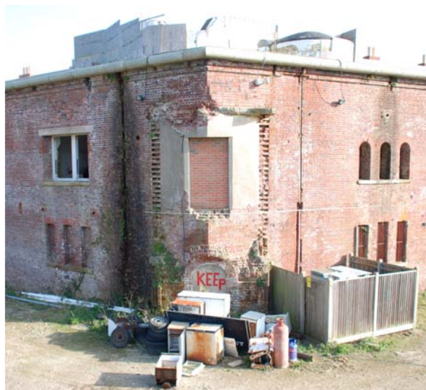
Image 36: Detail of upper storey: brick scars and concrete roof remnants.
