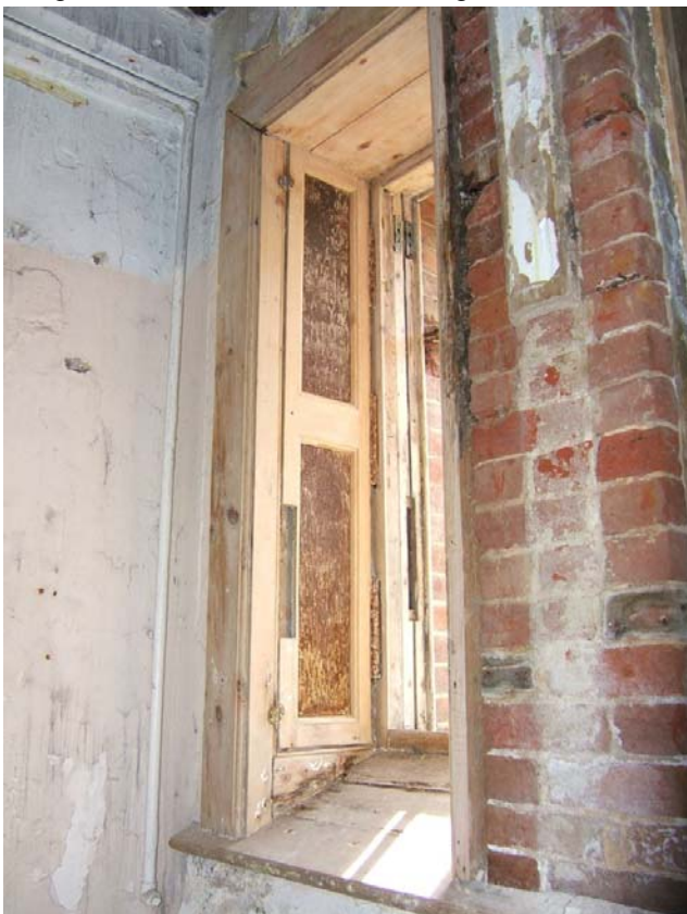
Image 61: Shutter in situ in wooden window frame.
