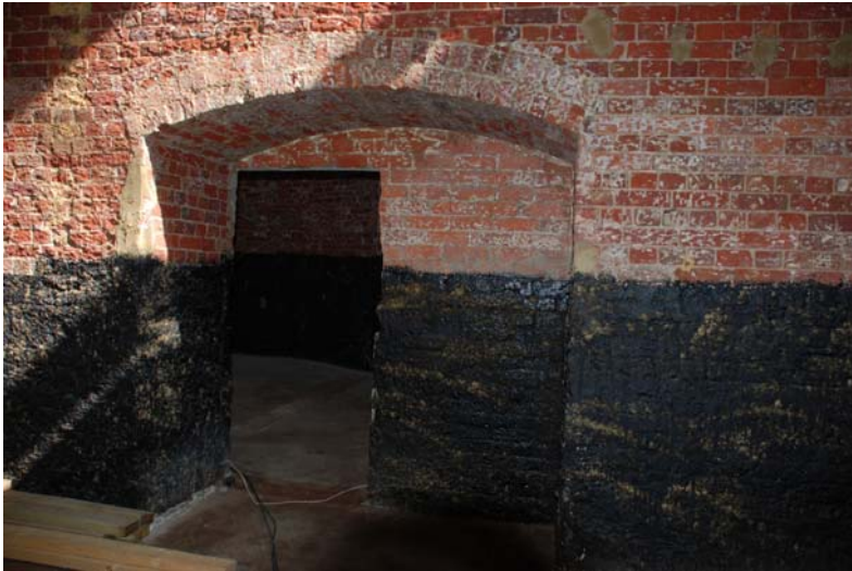
Image 37: Large original doorway, with later single skin brick infill and doorway. View from the tap room through to the canteen room.
