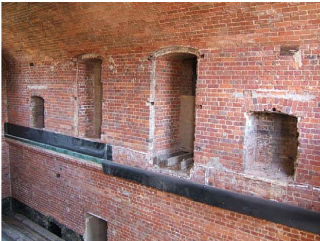
Image 55: First floor fireplaces showing hot air vent opening above.
