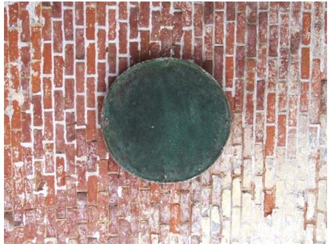
Image 54: Vent cover in place over vaulted ceiling of first floor barrack room.
