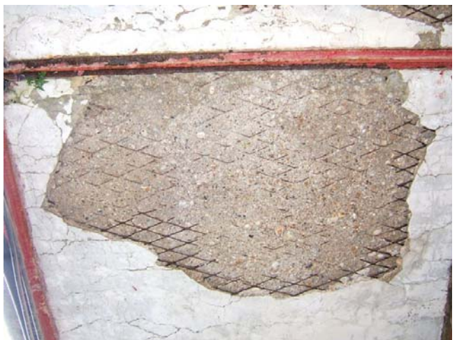
Image 14: Concrete floor of veranda. Floor of washroom was also of similar construction.
