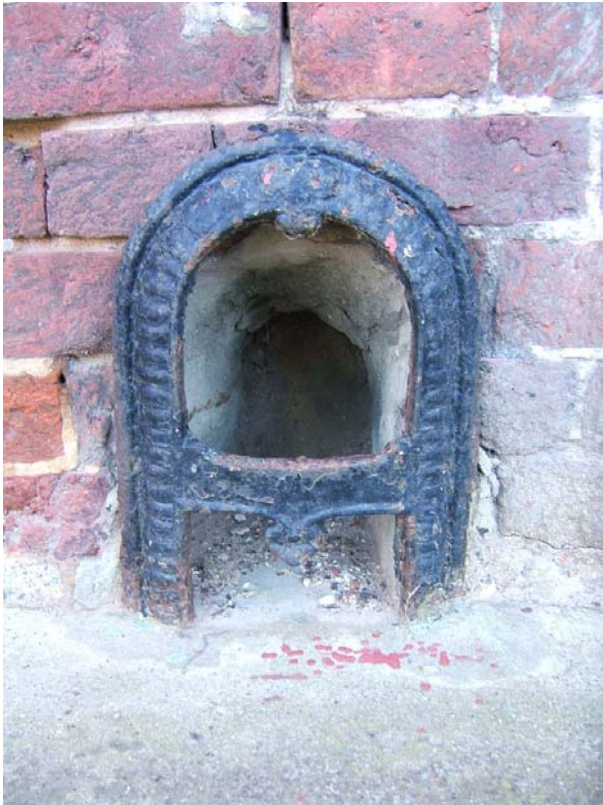
Image 71: Foot scraper outside ground floor barrack room.
