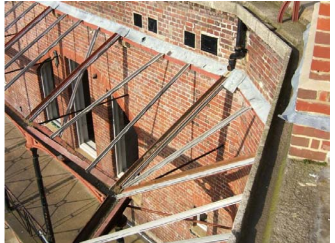
Image 70: Interior roof gutter and veranda roof structure.
