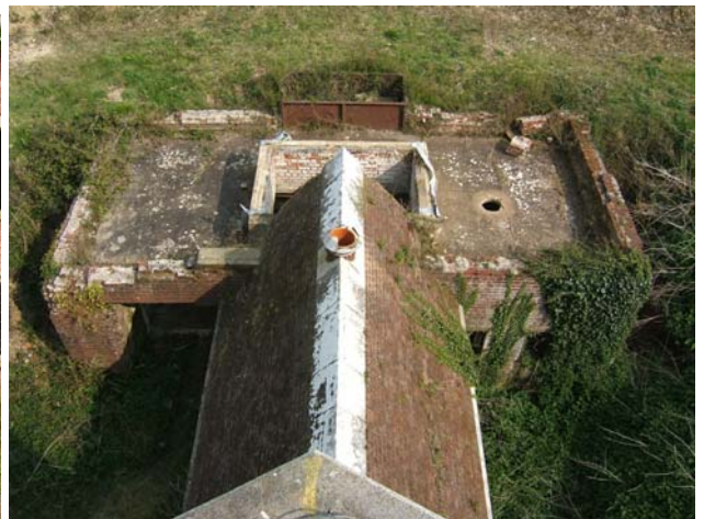
Image 12: Caponier from above, showing cast iron water cistern and roofless skylight.
