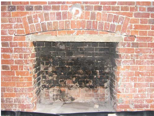
Image 21: Altered fireplace with insertion of sandstone lintel and brick infill.
