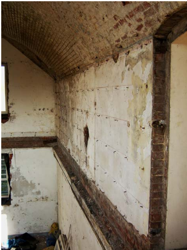
Image 39: Dry lining of barrack rooms. Batten nails and builders mark lines are visible.
