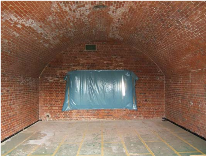
Image 01: Interior of barrack room showing vaulted brick ceiling.
