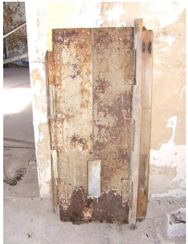
Image 62: Shutter arrangement with closed shutters showing loophole.
