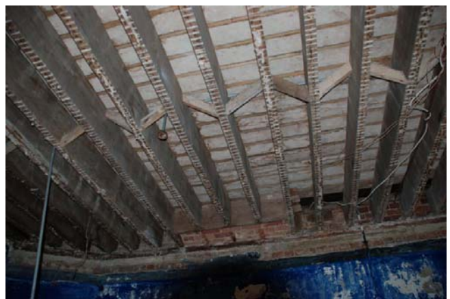
Image 52: Under floor bracing for first floor .
