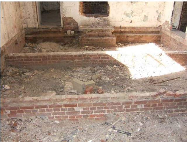
Image 83: Brick supports for ground floor wooden suspended floor.
