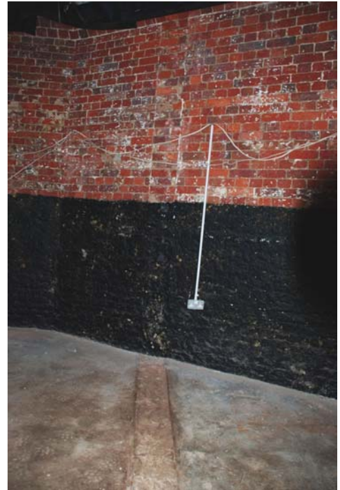
Image 38: Lobby to canteen room showing scars of removal of partition walls.
