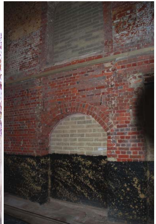
Image 44: Passageway in the married quarters on the ground floor with access blocked up.
