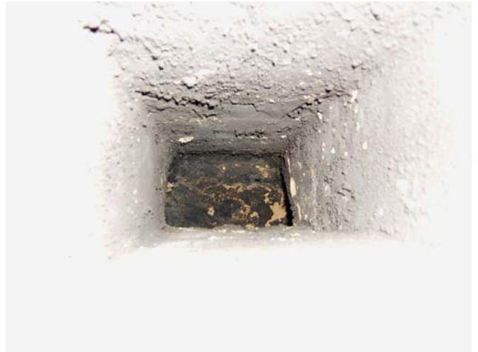
Image 20: Interior view upwards of vent in soffit of fireplace.
