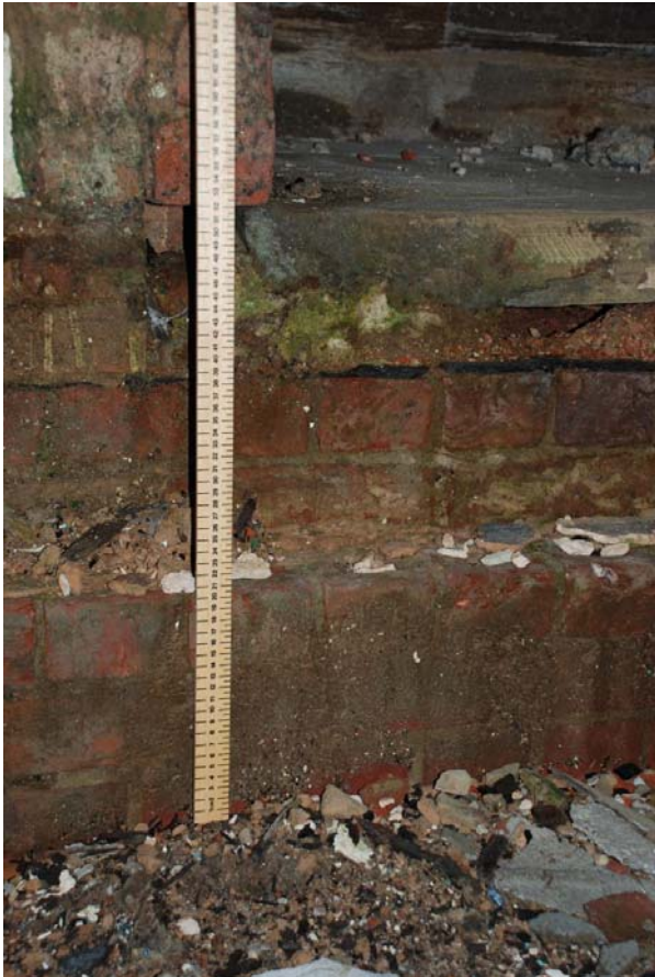
Image 63: Bitumen damp course on ground floor.
