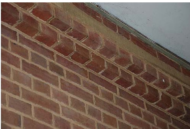
Image 51: Corbelling arrangement. This picture shows the ceiling of the entrance passageway.
