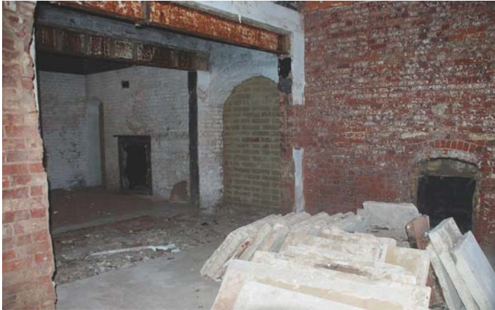
Image 41: View of original married quarters, showing infilled central passageway, running from left side to blocked doorway. Originally a wall existed either side of this passageway, with a door to allow access to the room either side, identified by the fireplaces. These two walls were demolished and replaced with an steel joist to allow more room for the later industrial units.
