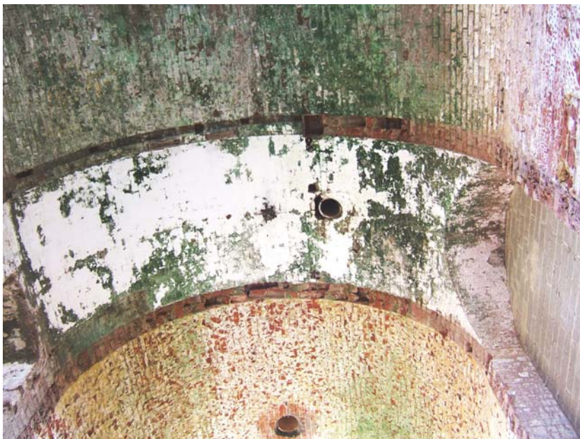
Image 43: View up to the roof of the first floor showing the scar marks of the original dividing walls for the married quarters. Blocked up access to passage can be seen on right. Vent holes in the vaulted ceiling are visible.
