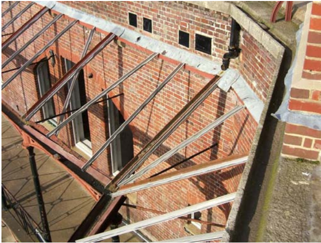
Image 09: Interior roof gutter and arrangement of down pipe with veranda.
