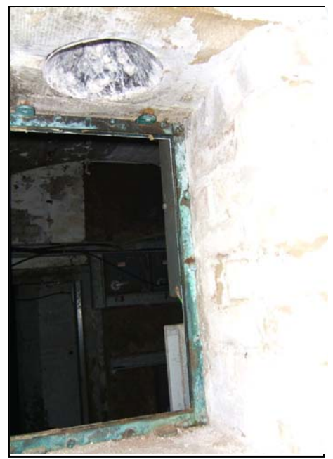
Image 78: View of the top of ammunition hoist showing iron ring for hoist tackle.
