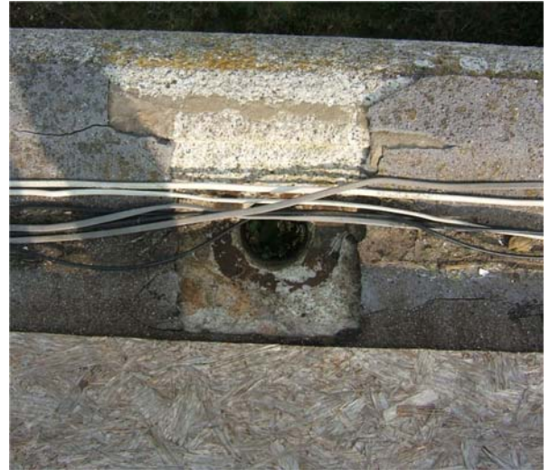
Image 02: Aerial view of roof coping showing asphalt layer.
