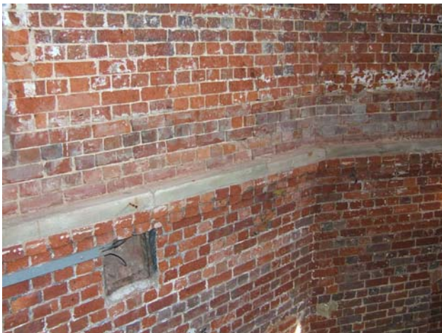
Image 07: Brick corbelling of first floor with sandstone plinth.
