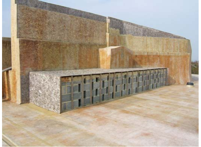
Image 10: Cistern on roof. Originally cast iron, now screened off with block wall.
