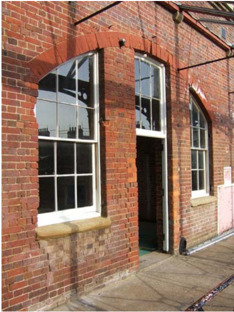
Image 15: Original entrance to a barrack room, showing door and window arrangement.
