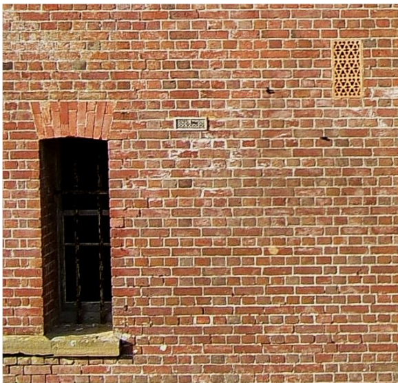
Image 17: Exterior wall of fort, showing coverings for internal vents.
