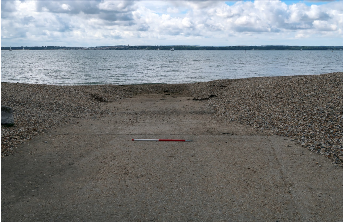
Figure 58. Post-war concrete slipway at the western end of Stokes Bay, scale 1m (© Historic England).
