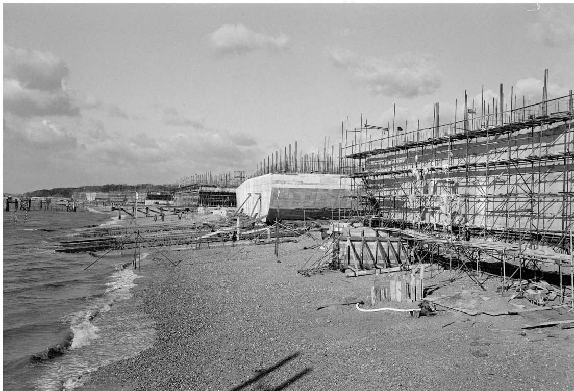
Figure 9. Phoenix caissons under construction at Stokes Bay, 1944 (copyright Imperial War Museum, H 35554).
