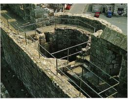
The cistern, on top of the aptly named Cistern Tower, collected rainwater from the adjacent roofs. Surplus water could be fed by a system of channels to an outlet in the Queen's Gate.
