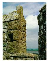
A section of the battlements on top of the Watch Tower showing one of the grooves in which a wooden shutter was hung for the protection of crossbowmen.
