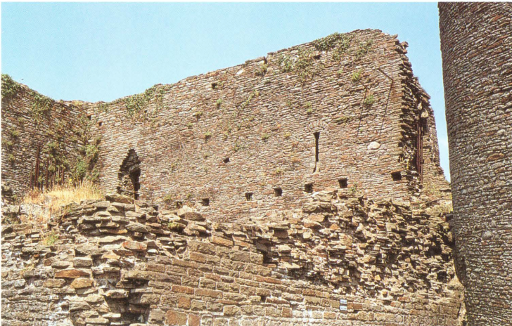
Looking carefully at the southern curtain wall of the inner ward, it is possible to find traces of arrowslits and beam holes at two levels. The curtain wall was raised in height and a stone-vaulted passage — the Braose Gallery — created within its thickness.
