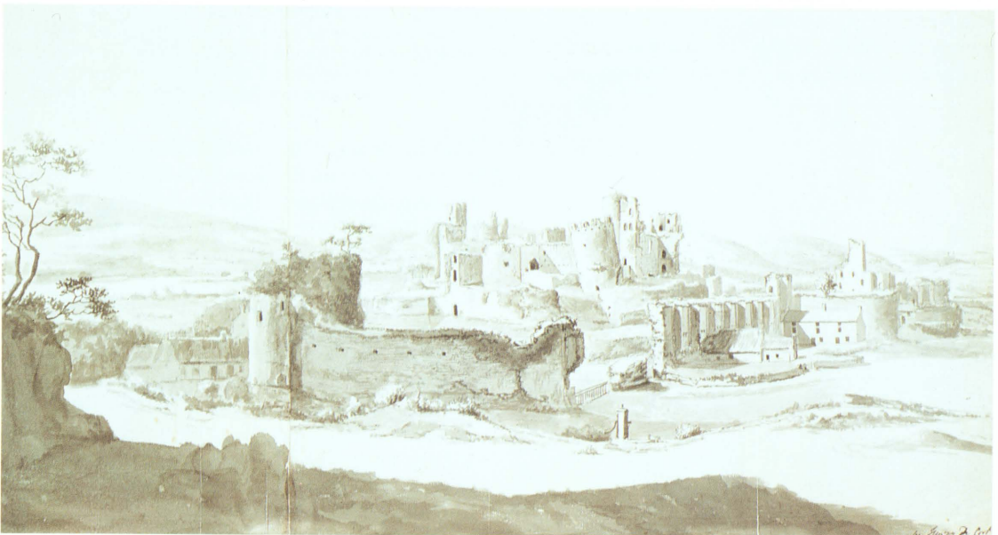
During the later Middle Ages, Caerphilly Castle appears to have been allowed to fall into gradual decay. By the time Henry de Cort (1742–1810) produced this watercolour in 1793, the front of the east gatehouse had already collapsed, the south-east tower was leaning, and there was a large breach in the south dam (By courtesy of the National Library of Wales).
