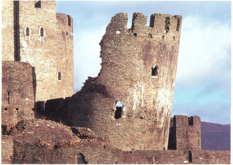
Caerphilly's most celebrated feature is perhaps its 'leaning tower', the south-east tower of the inner ward. It leans at an angle of 10 degrees, probably the result of ground subsidence.
