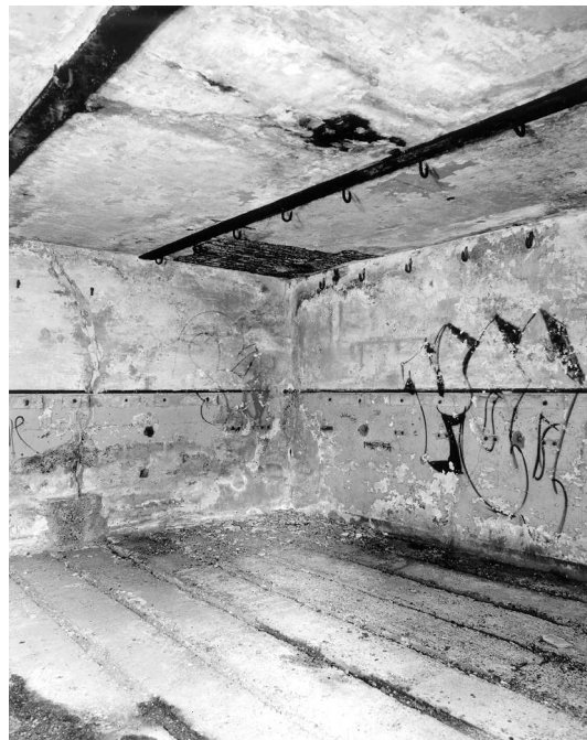
Figure 11 The interior of the Men's Shelter showing hammock hooks in the ceiling (NMR: AA98/07906)
