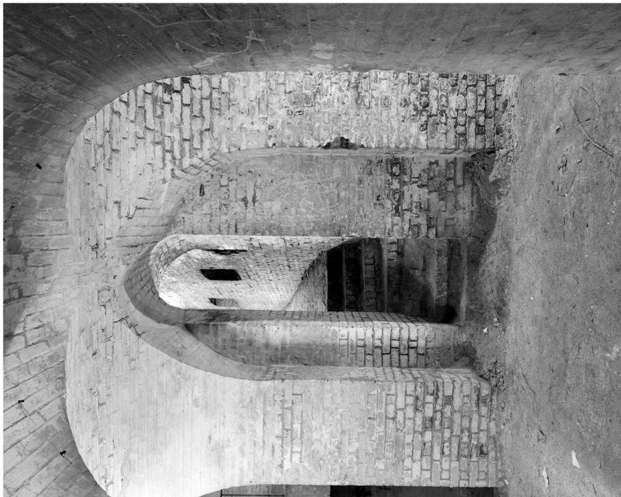
**Figure 31:** Detached Bastion; photo of the entrance to the west musketry gallery upper floor, viewed from the rear of the north-west caponier, showing elaborate brick vaulting (NMR: AA008636 © Crown Copyright 1998)
