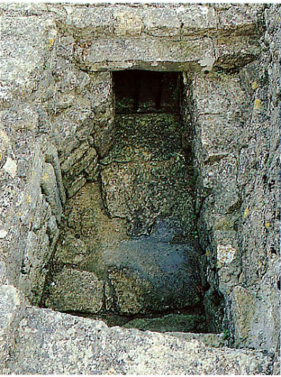
Above: The main drain of the inner court of the castle. Within the drain is a groove for a wooden sluice that could be raised and lowered to regulate the flow of water
