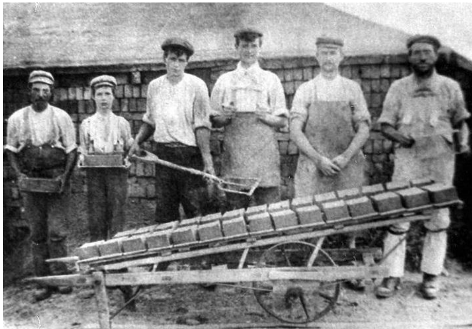
A brickmaking gang at Rainham in 1890 standing in front of a hack. Note the moulds, large cuckles and brick barrow.
