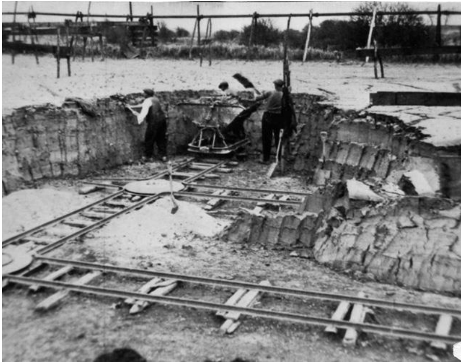
Excavating a washback in one of the larger Eastwood brickfields in the 1900s. The slurry launders can be seen in the background.
